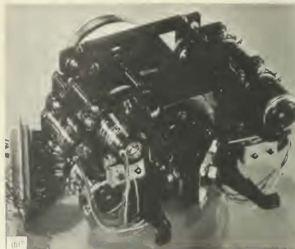
FIGURE 3-4.—Lens assembly of the Surveyor television camera. (a) Front view. (b) Back view.
