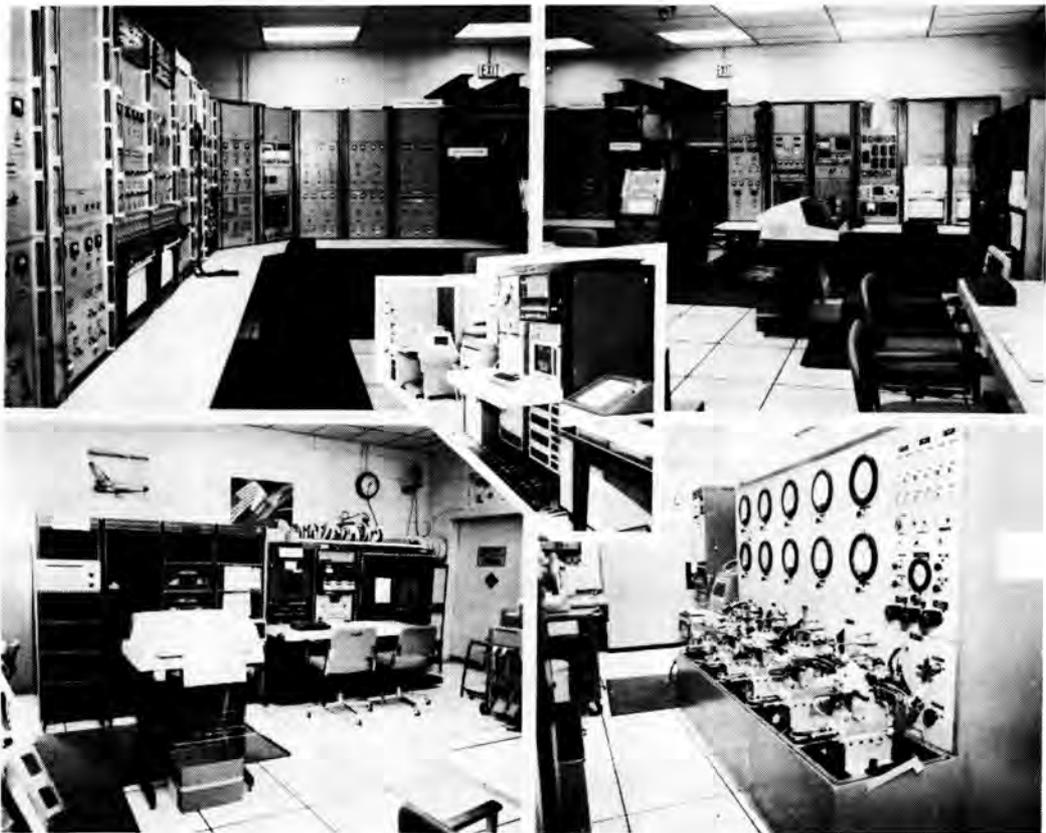
Figure 9-4. A collage depicting the Hardware Simulation Laboratory at the Marshall Space Center used for testing the Shuttle Main Engine Controllers. (NASA photo 331594)
