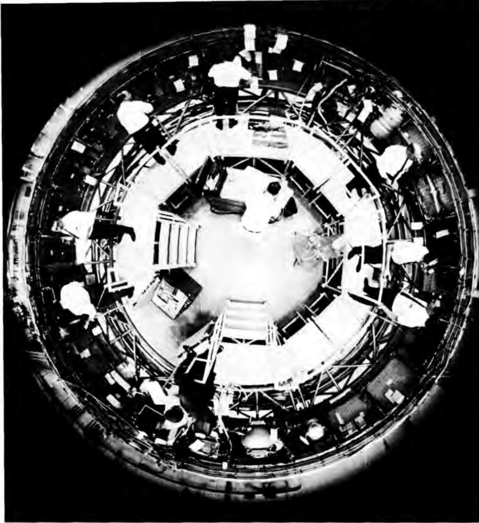
Figure 7-2. IBM engineers work inside the Saturn launch vehicle Instrument Unit. (IBM photo)
