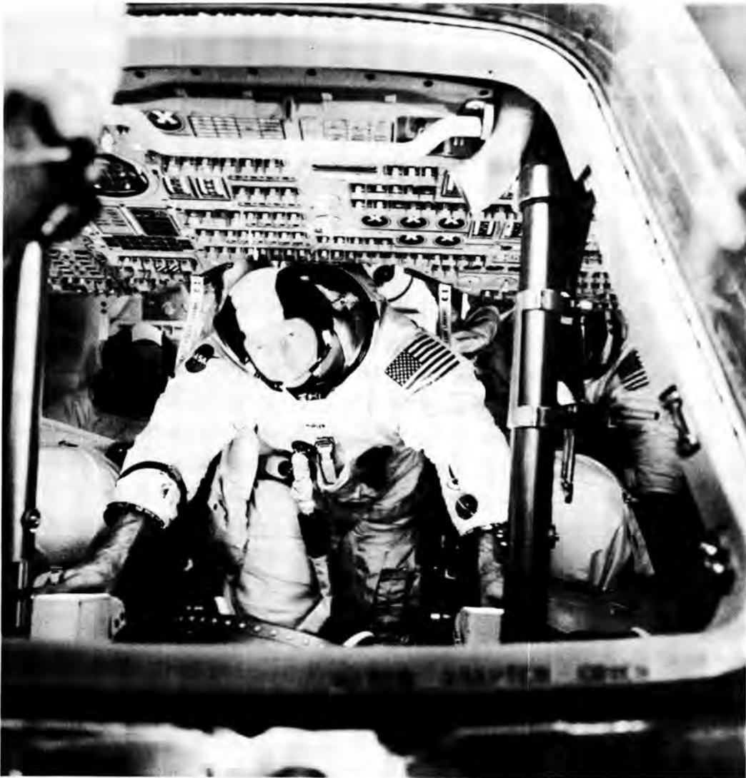
Figure 2-4. The interior of an Apollo Command Module, showing the location of the DSKY on the main control panel at the left. Apollo 15 crewmen shown include Alfred M. Worden (center) and David R. Scott (left). James B. Irwin is mostly obscured to the right. (NASA photo S-71-29952)
