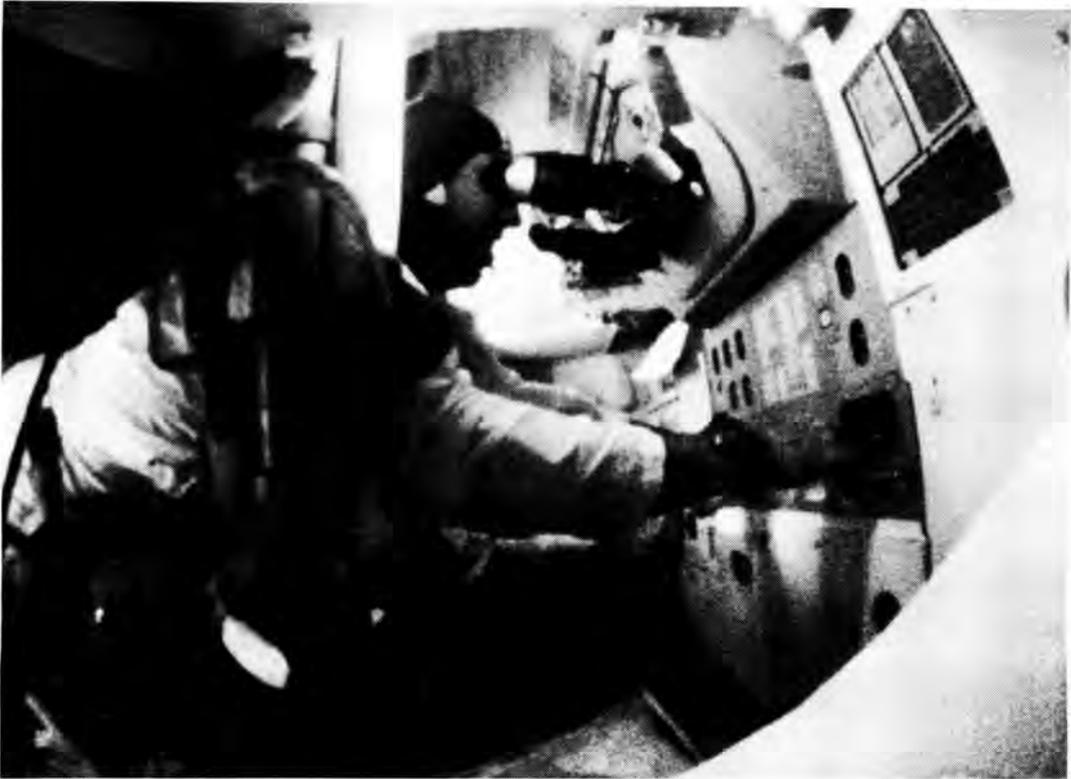
Figure 2-3. Another DSKY was located at the navigator's station in the command module. Astronaut James A. Lovell takes a star sighting during the Apollo 8 mission. (NASA photo S-69-35099)
